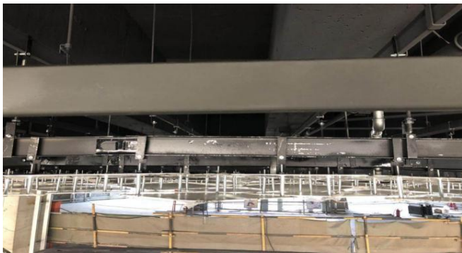
图2 双层主龙骨安装示意
